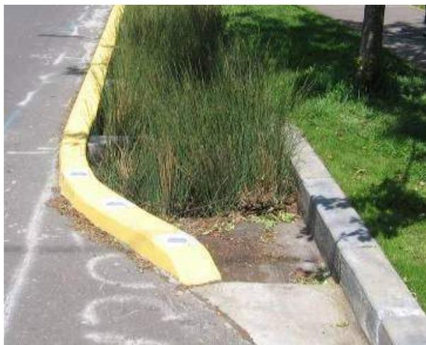
**Figure 9-A.3. Stormwater Curb Extensions**
