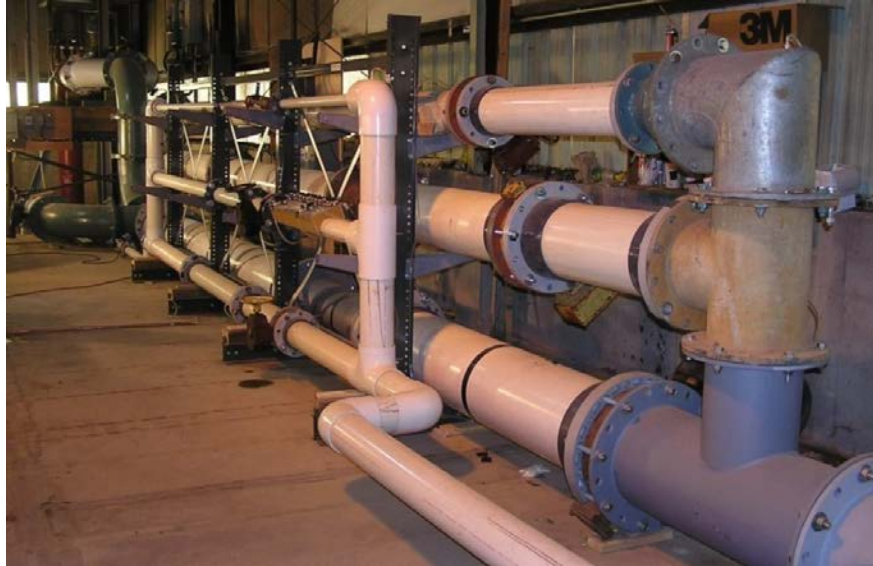
Figure 5 Photograph Showing Laboratory Flow Meters
