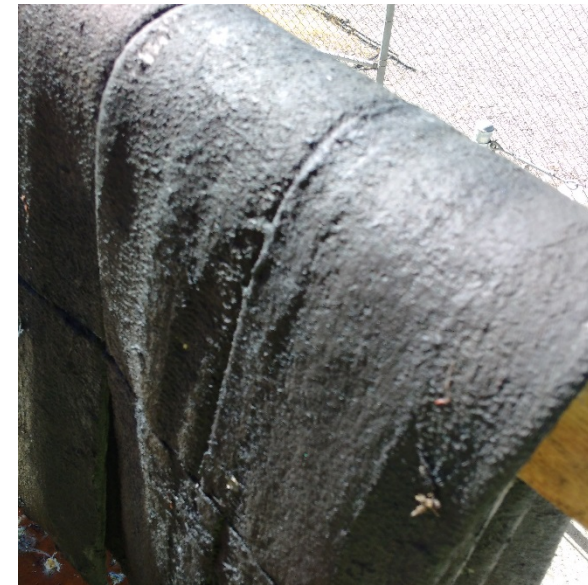
Sediment build up on filter Ribbons
