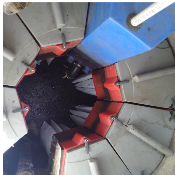
Newly installed filter Ribbons
