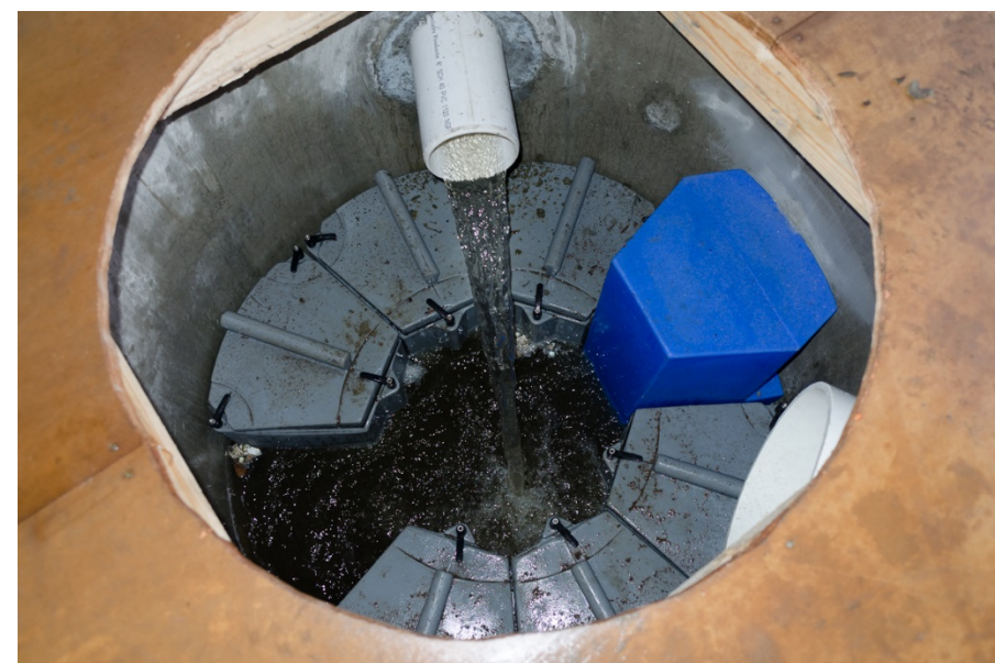
Filter modules during storm event
