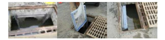
In the case of only floatables removal, a vacuum truck is not required. However, a vacuum truck is required if the maintenance event is to include oil removal and/or sediment removal. Proof of inspections and maintenance is the responsibility of the owner. All inspection reports and data should be kept on site or at a location where they will be accessible for years in the future. Some municipalities require these inspection and cleaning reports to be forwarded to
