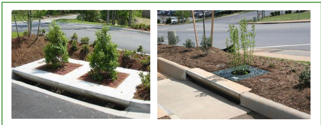
Figure 1. Typical Filterra System Application.
