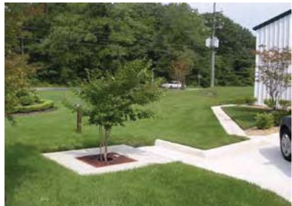
High flows bypass Filterra into a grass swale.
