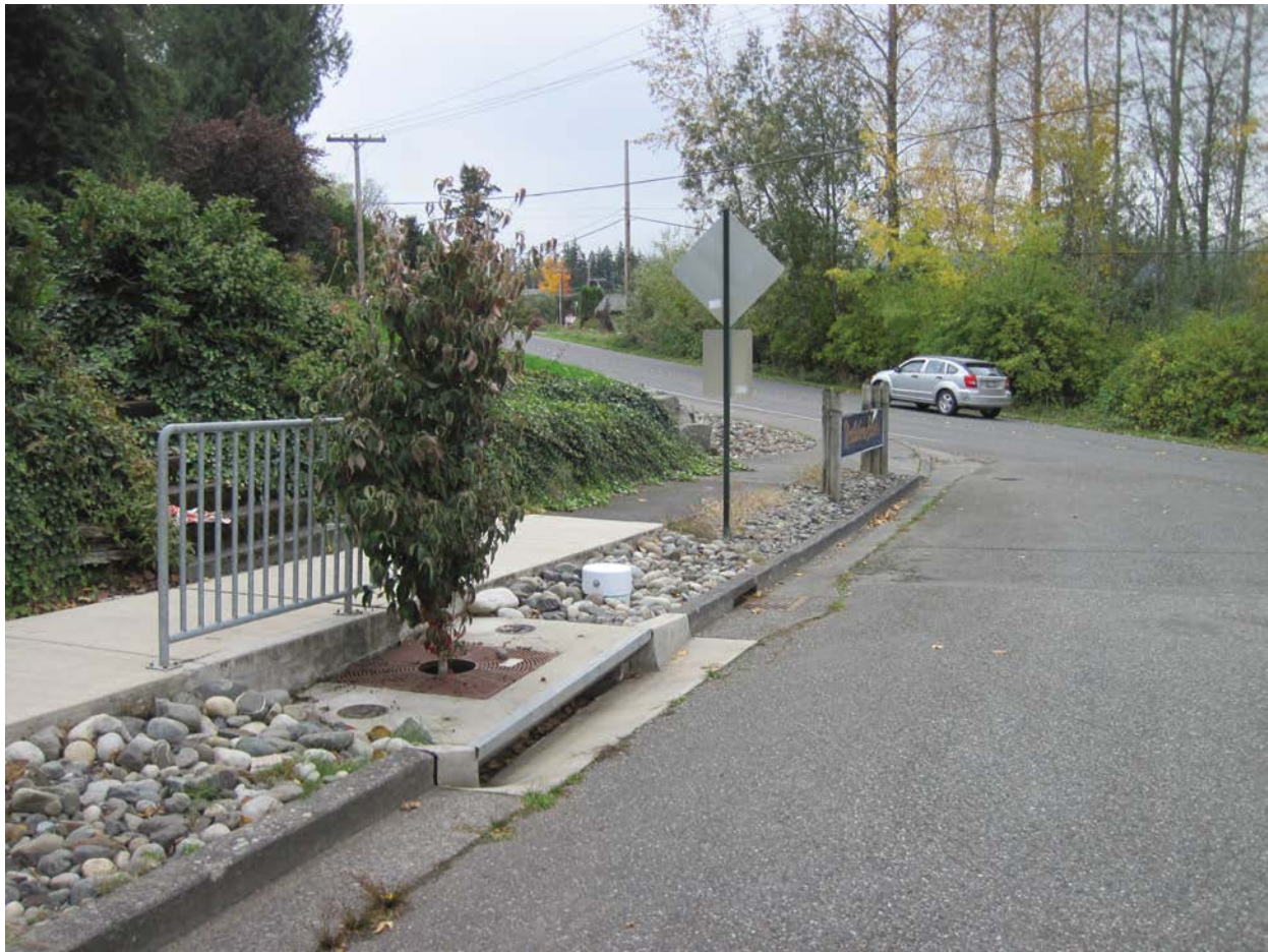
Figure 4. Photograph of the Hayward Drive Filterra system.
