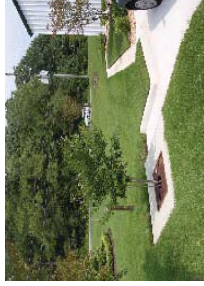
High flows bypass Filterra into a grass swale.
