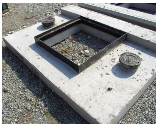
Modified recessed top prior to shipping
