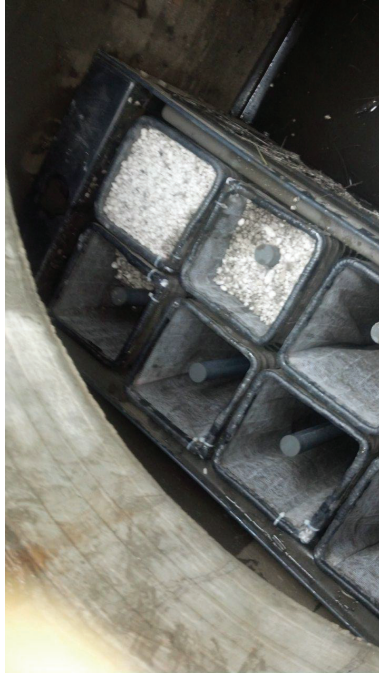
Installation of temporary perelite prefilter with new cartridge design
