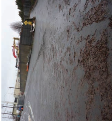
High sediment loading in drainage basin
