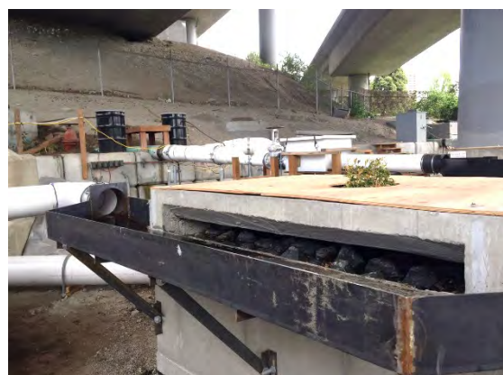
Installation of the monitored StormGarden™ system at the Ship Canal Test Facility in Seattle, Washington.
