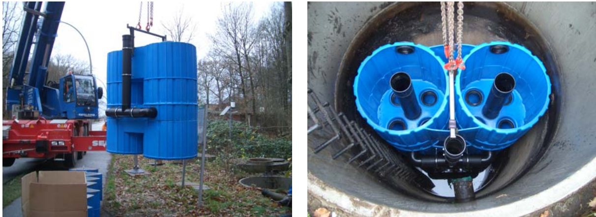
Figure 2. The installation of the system.
