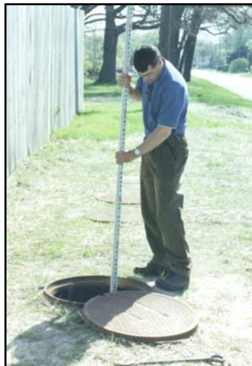
Sediment inspection using a stadia rod
